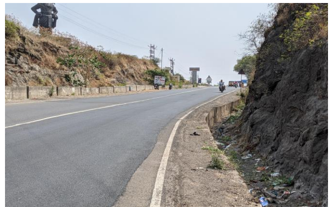
Image -1: Open Side Drain and no shoulder
