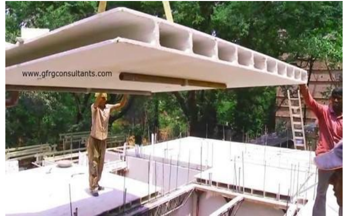
Roof panel installation
