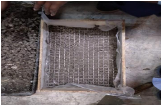
Fig. no. 10 Placing of Galvanized steel weir mesh
