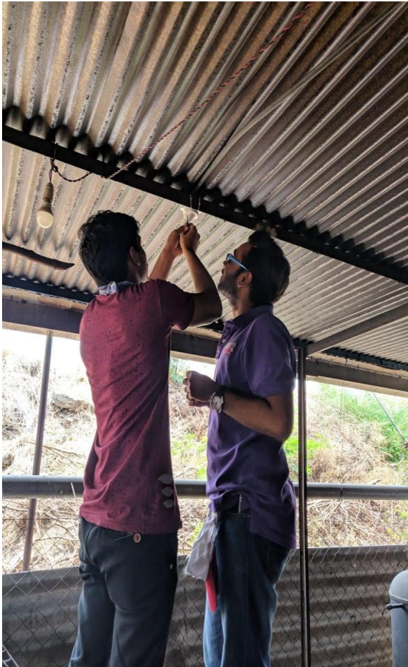
FIGURE 6:- INSTALLATION OF DC LOAD
