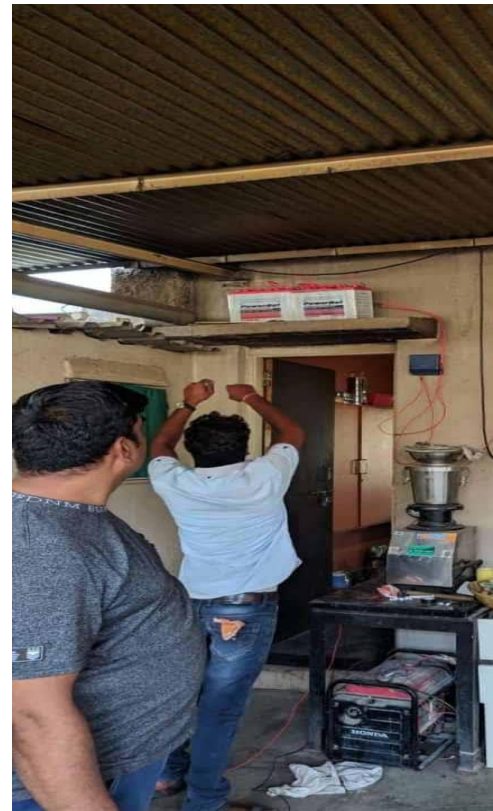
FIGURE 5:- INSTALLATION OF BATTERY BACKUP
